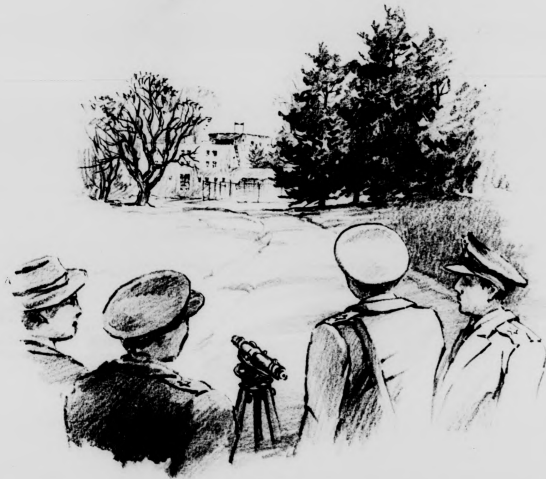
Figure 3 - General view of experiment on roof as seen from observing station 900 feet distant.
